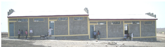
Front elevation with the entrances to the four classrooms. Fourth from left: Gerard Versteegh.
